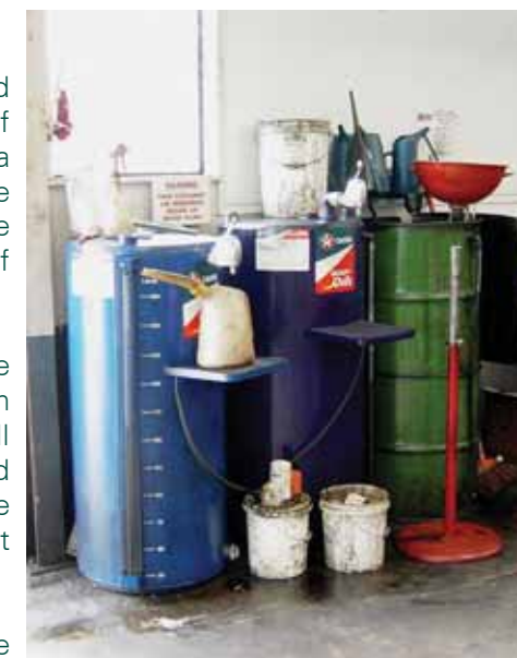
Oil store before 'bunding'
